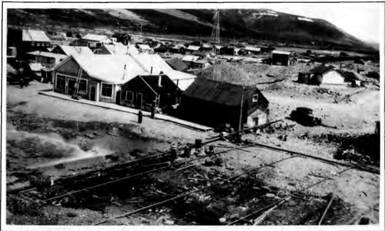
Figure 8. The Donnelley and Sheppard complex, including the Store (left), Assay Building (center) and Standard Oil Warehouse (right), 1930. Photo courtesy of John Miscovich, Flat, Alaska.
